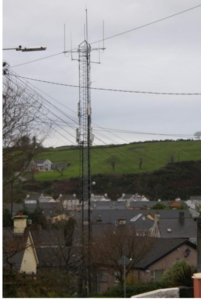
Transmitter Site Photo
